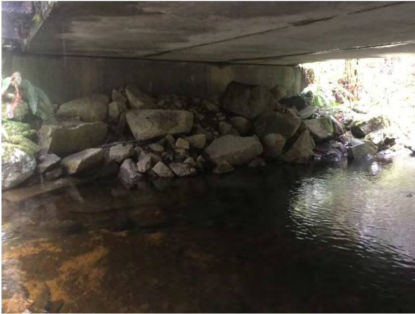
Right Bank Abutment when facing downstream
