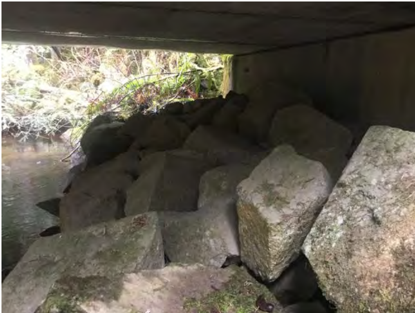
Left Bank Abutment when facing downstream
